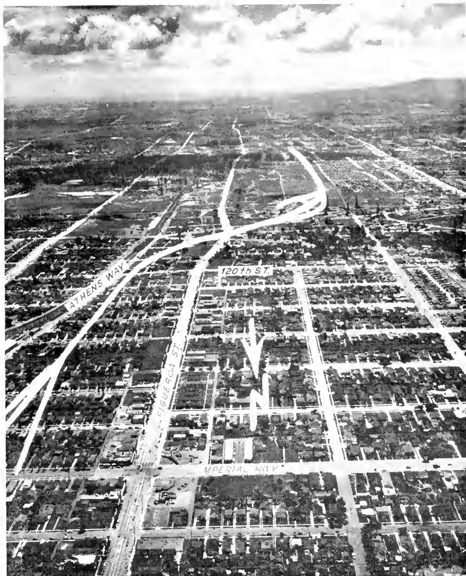
Looking southerly along route of Harbor Freeway, showing Los Angeles Harbor in background, left, and Palos Verdes Hills background, right. The curving location of the Harbor Freeway that was necessary in order to miss highly productive oil wells is shown.
